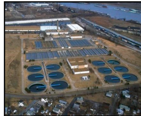
Lemay Treatment Plant
